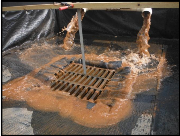
Figure 11. Inlet Filter Bag Testing
