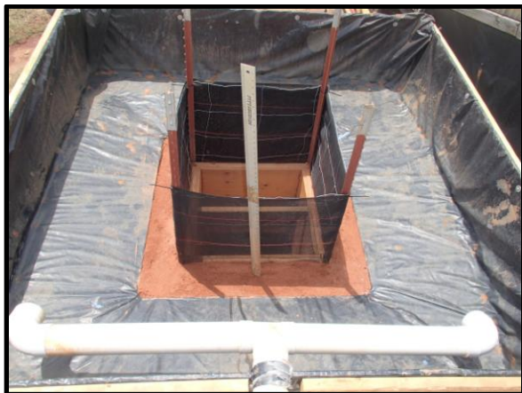
Figure 8. Silt Fence on Support Posts with Welded Wire Fencing (WWF)
