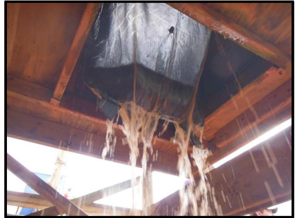
Figure 12. Inlet Filter Bag Close-up
