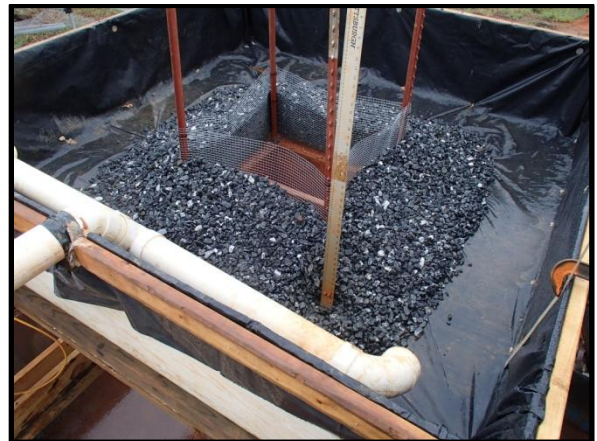
Figure 5. Stone and Wire Mesh backing
