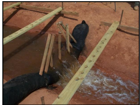
Figure 10. Testing of a Compost Sock Check Structure
