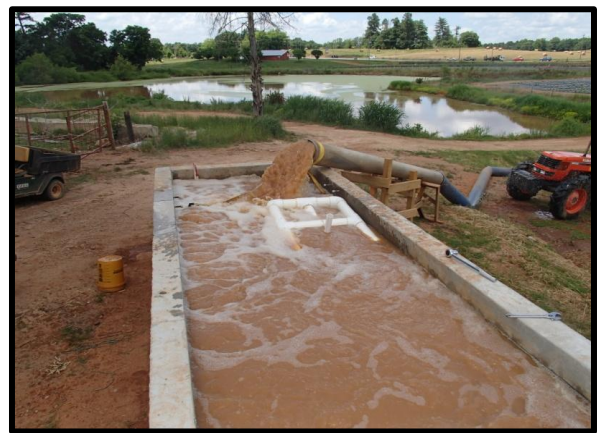
Figure 9. Skimmer Floats to Top during Filling
