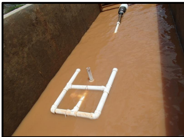
Figure 8. Skimmer Connected to Outlet Pipe via Flex Hose
