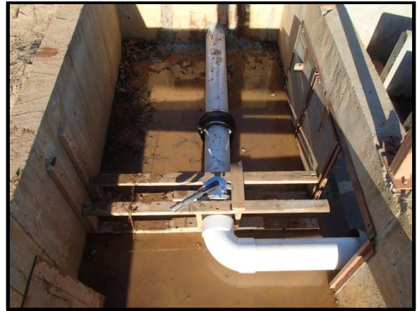
Figure 7. Outlet is Controlled with 8-inch Valve
