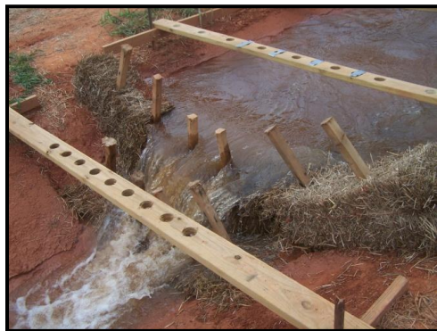
Figure 6. Straw Bale (NRCS) Check Structure
