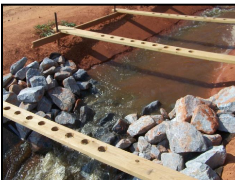
Figure 7. Rock Check Structure
