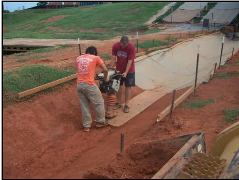
Figure 3. Compaction of Veneer
