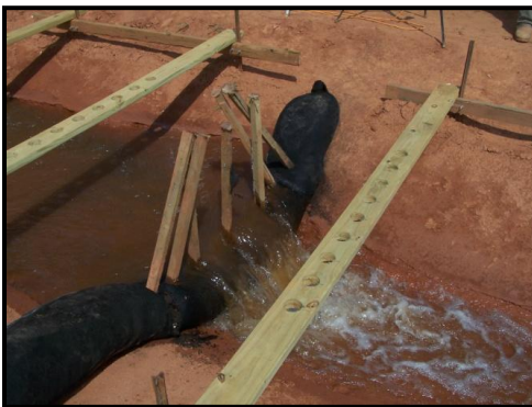
Figure 5. Compost Sock Check Structure
