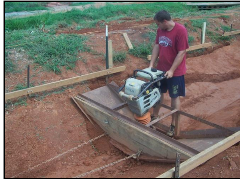
Figure 4. Channel Forming (typical)
