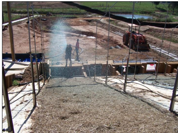
Figure 3. Tackifier Being Applied to Straw
