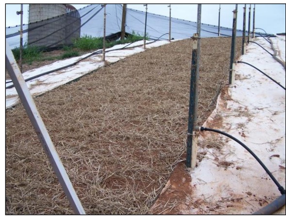
Figure 6. Straw Crimped into Slope
