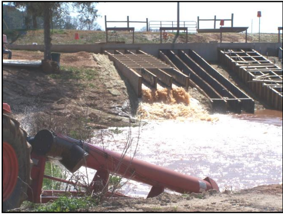
Figure 1. Typical 10% (Unvegetated Shear) Flumes on Left; 20% Flumes on Right
