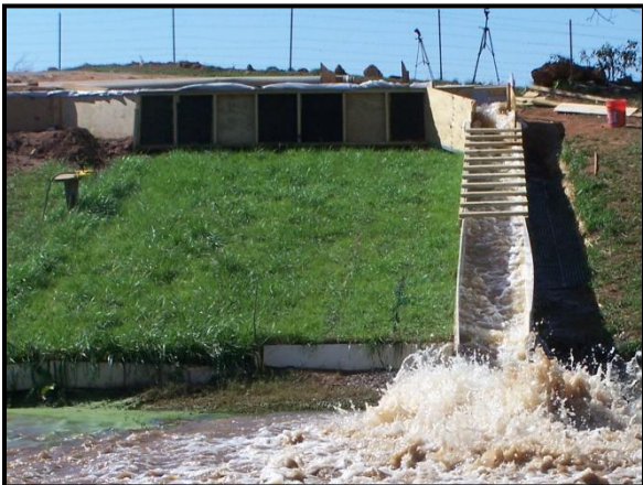
Figure 3. Typical 20% Temporary Flume Set Up 1+ Year Vegetated Shear Plots
