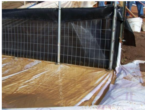
Figure 11. Silt Fence #4 + Wire Backing
