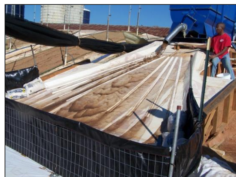
Figure 8. Silt Fence #1 + Wire Backing
