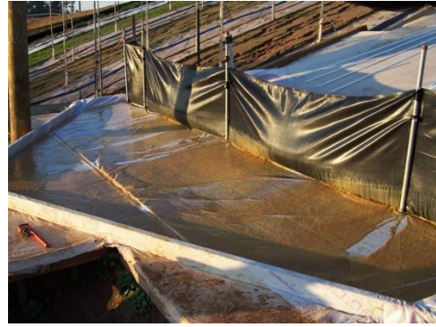
Figure 10. Silt Fence #3
