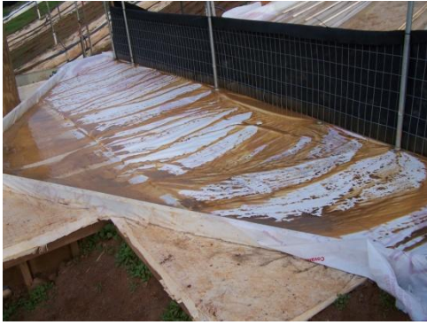
Figure 9. Silt Fence #2 + Wire Backing
