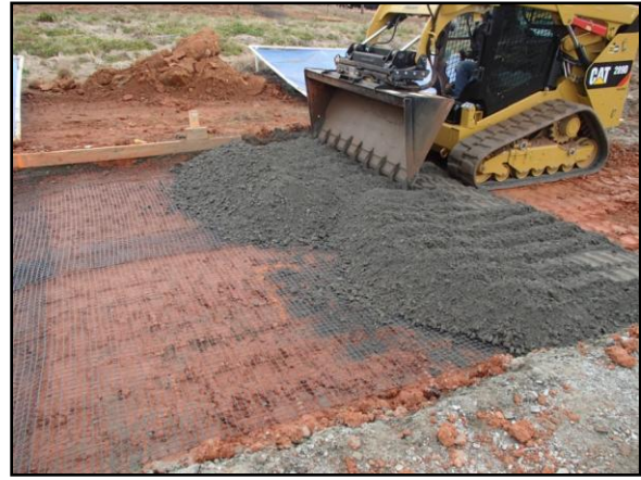
Figure 4. Geogrids Positioned and Covered with Based Aggregate
