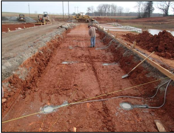
Figure 3. Installation of Pressure Cells
